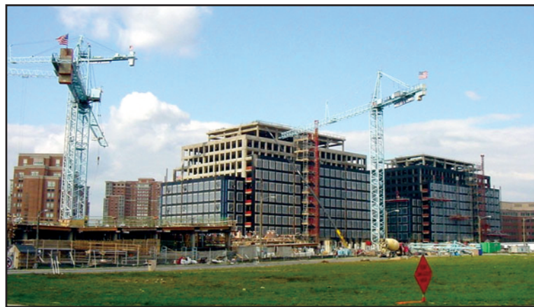
On the left is the Jefferson Building, like the Remsen Building, it is scheduled for occupancy in December 2003.
