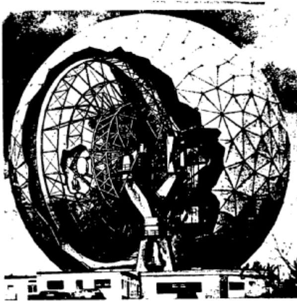
Fig. 1. M.I.T. Haystack Observatory's 120-ft parabolic antenna enclosed in 150 ft MSF radome.
